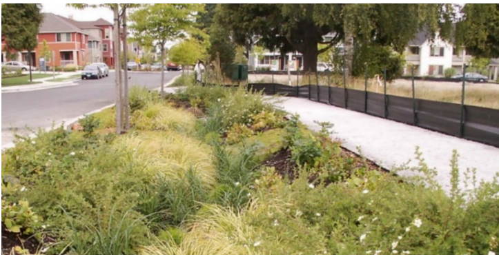
Examples of natural drainage systems a few years after installation
